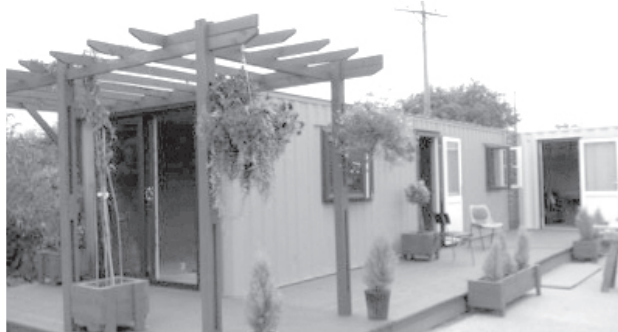
Howell's 2018 Container “show house”. Builder's yard, Bridgwater Somerset. http://robinhowell.org/project-diary-2/
